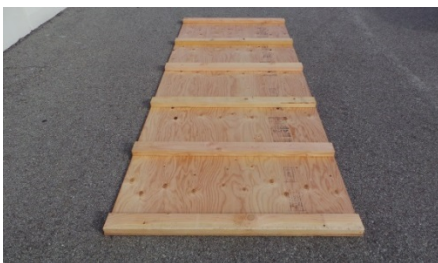
Separate 2x4s approximately 20" apart from each other (20" centers).
