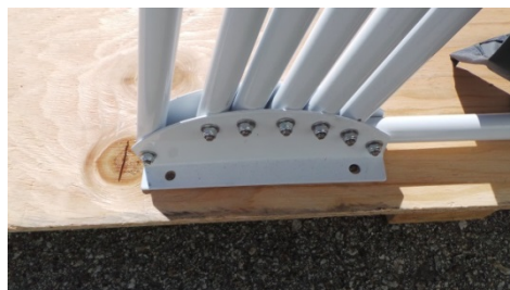
Locate 2-each anchor holes on both sides of the frame assembly. Mark and drill the holes.
