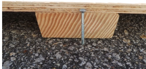
Attach 2x4s to plywood using 2 inch woodscrews.
