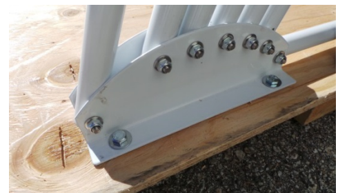
Secure the frame to plywood using 1.5" bolts, washers, and nuts.
